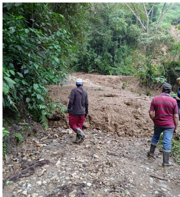
Damaged roads in Tolima
